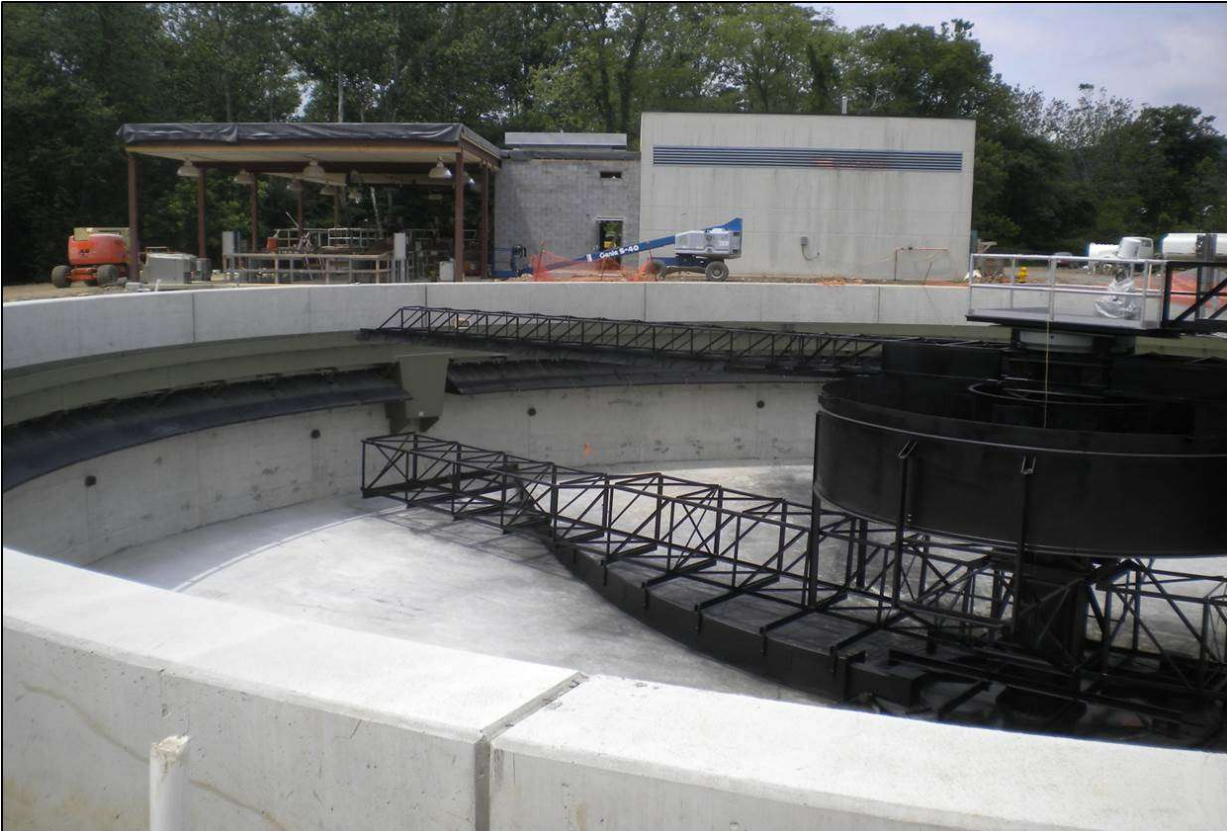
Figure 10.26 Final clarifier for an activated-sludge secondary with rapid-sludge-removal apparatus. (Courtesy of Dorr-Oliver, Inc.)
